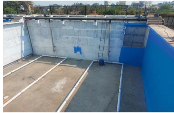
STP under construction – Aeration Tank (SBR basin)
