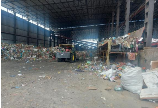
Inside view of RDF and Compost Plant with Material Recovery Facility, Pune
