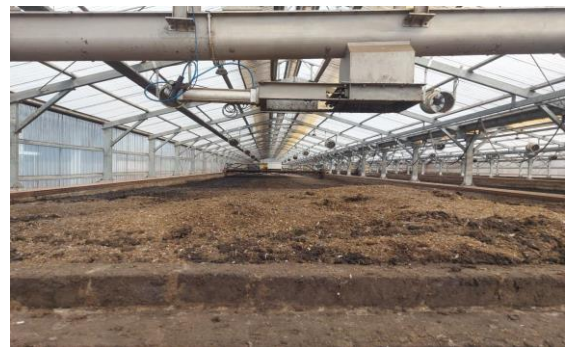
Composting of Wet Waste at Saligaon, Goa
