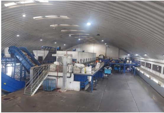
Dry Waste Micro Segregation facility at Saligaon, Goa
