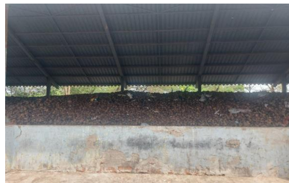
Coconut Storage Shed – Saligaon, Goa
