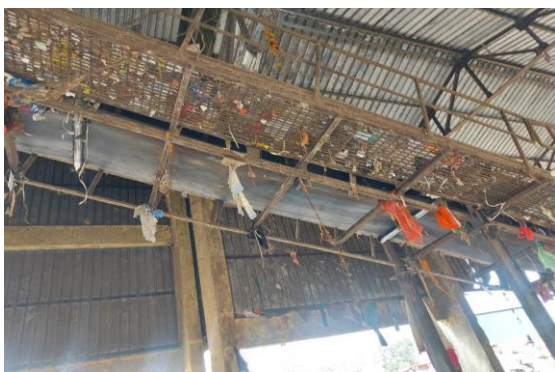
Material Recovery Facility (MRF)
