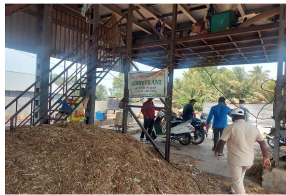
20 TPD slurry plant
