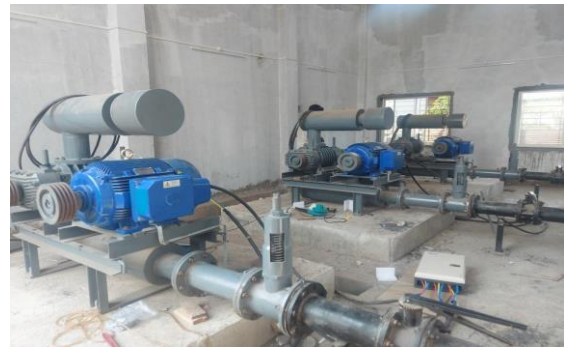
STP under construction – Blower Room
