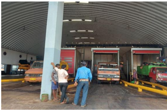
Unloading of Wet Waste, Saligaon, Goa
