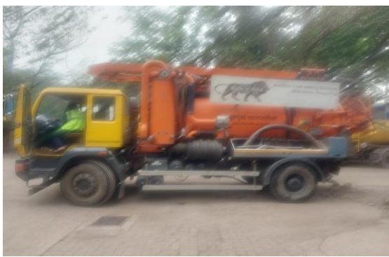
Plate 5 : Mechanical Cleaning System - Sewers
