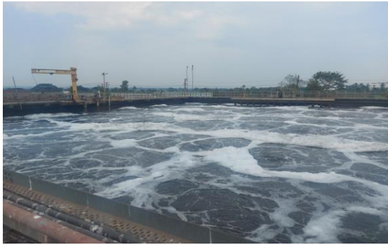
STP Aeration Tank ( C-Tech Basin)
